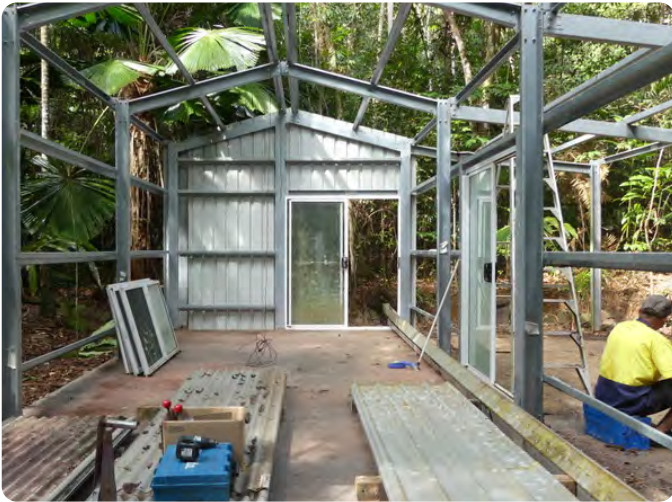
Disassembly of the Barratt Creek shed. Image: Barbara Maslen
