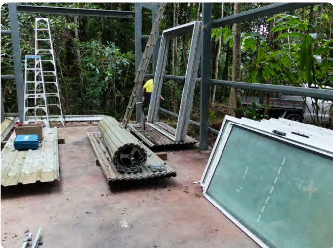
Windows, sliding doors will all be repurposed. Image: Barbara Maslen
